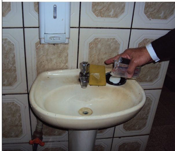
FIGURE 9 Personnel hygiene facility in a bad condition. Facilities should be clean, with a supply of potable water, liquid soap and means for drying hands
