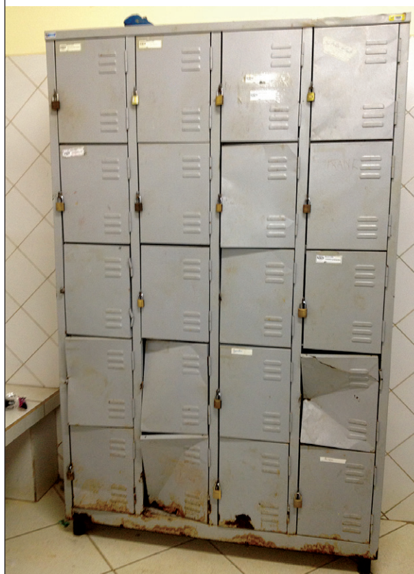
FIGURE 10 Lockers for personnel items in a bad condition. Not in accordance with GMP
