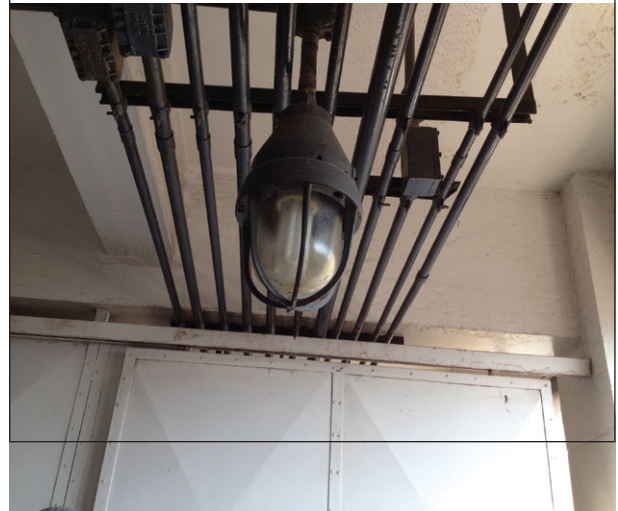
FIGURE 13 Light well protected
