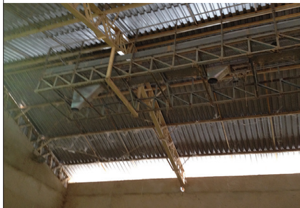
FIGURE 8 Openings in the ceiling allow the entry of pests, birds and dust that can contaminate the production environment
